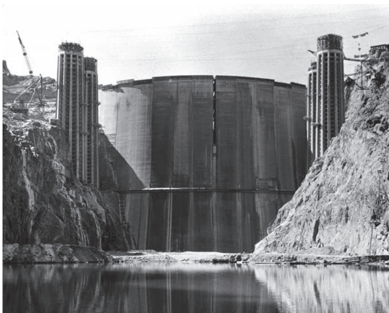
Fig. 3.1 Construction of Hoover Dam (1931–1935) on the Colorado River. For many years the largest dam in the world, Hoover Dam was constructed to meet irrigation needs and provide flood control and electric power for the southwestern USA. (From US Bureau of Reclamation)
