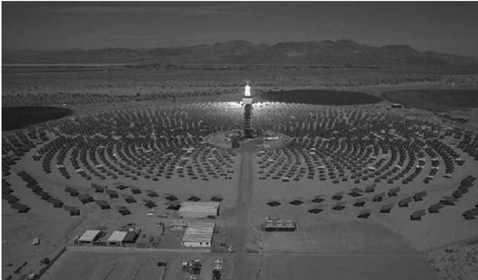
Figure 13.30 “Solar Two” central receiver plant.
