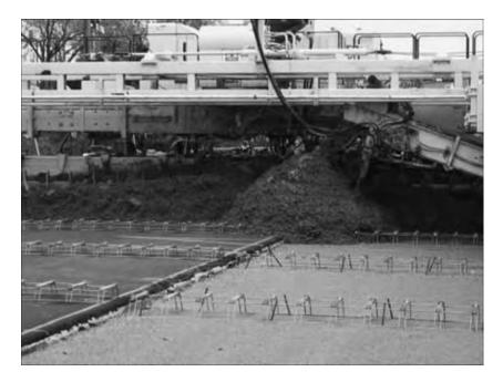
Figure 18.3 Unbonded overlay on two lanes with a third lane paved at the same time (photo courtesy: Dale Crowl).
