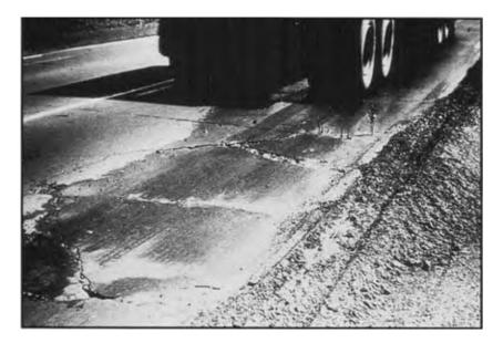
Figure 3.11 Water bleeding and pumping (Miller and Bellinger 2003: 58).
