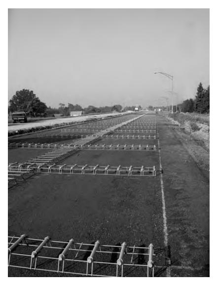
*Figure 1.1* Dowel and tie bar baskets placed in preparation for slipform paving (photo courtesy of The Great Lakes Construction Company, Hinckley, Ohio).
