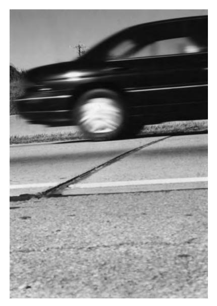
Figure 3.10 Faulted transverse joint (photo by author).
