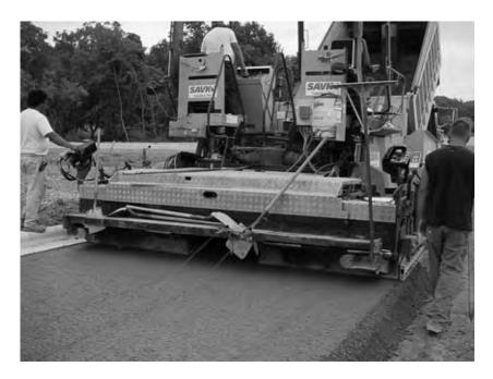
Figure 2.10 RCC pavement construction - Columbus, Ohio (photo by author).
