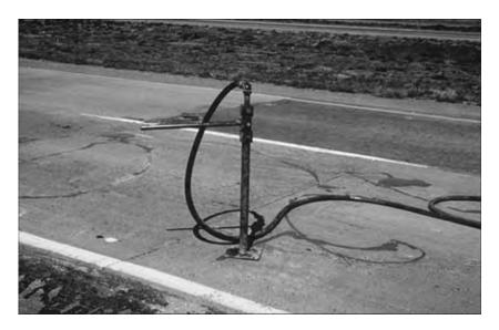
Figure 17.6 Grout injection for slab stabilization (ACPA 1996a: VIII-23).
