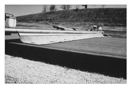
Figure 15.2 Burlap drag to provide microtexture (ACPA 1996a: VI-53).
