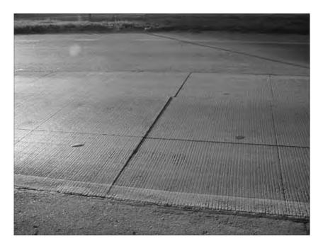
Figure 18.9 Failure of UTW by panel sliding (photo by the author).
