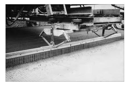
Figure 15.1 Transverse tining to provide macrotexture (ACPA 1996a: VI-53).
