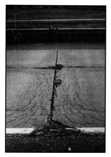
Figure 3.2 High severity D-cracking (Miller and Bellinger 2003: 37).
