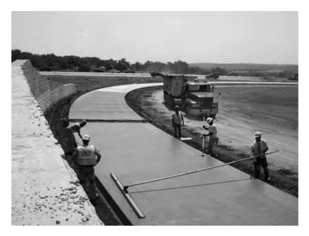
Figure 1.3 Finishing slipformed pavement around a banked curve (photo courtesy of The Great Lakes Construction Company, Hinckley, Ohio).
