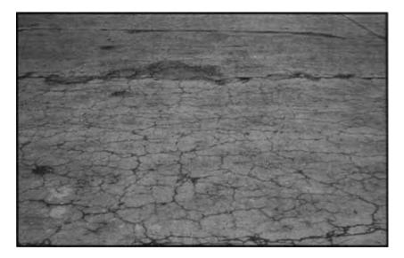
Figure 3.6 Map cracking (Miller and Bellinger 2003: 48).
