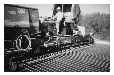
Figure 14.8 CRCP steel installation with tube feeders (ACPA 1996a: VI-37).
