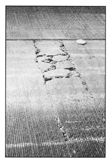
Figure 3.12 High severity punchout (Miller and Bellinger 2003: 79).
