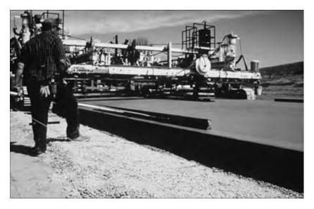
Figure 14.2 Concrete pavement produced by slipforming (ACPA 1996a: VI-6).
