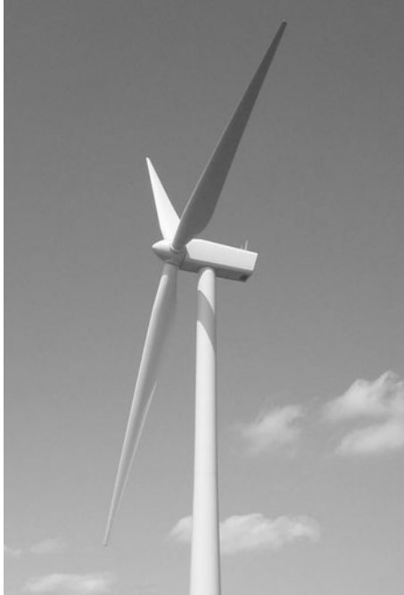
Figure 5.1 A typical modern wind turbine.
