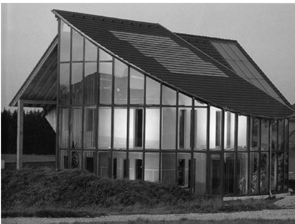
Figure 12.3 Solar low-energy building in Upper Austria.
