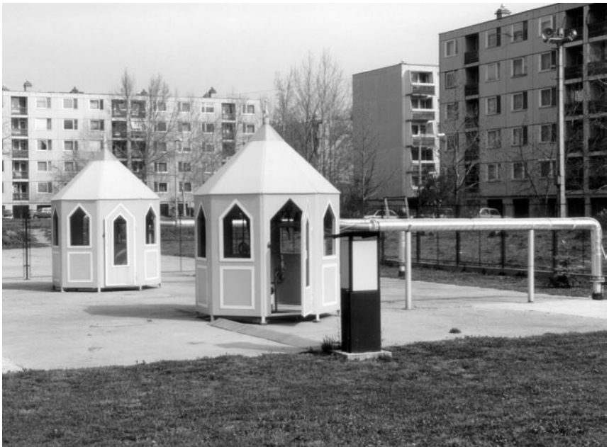
Figure 3.7 Two wells in Hungary supplying heating water to a housing complex.
