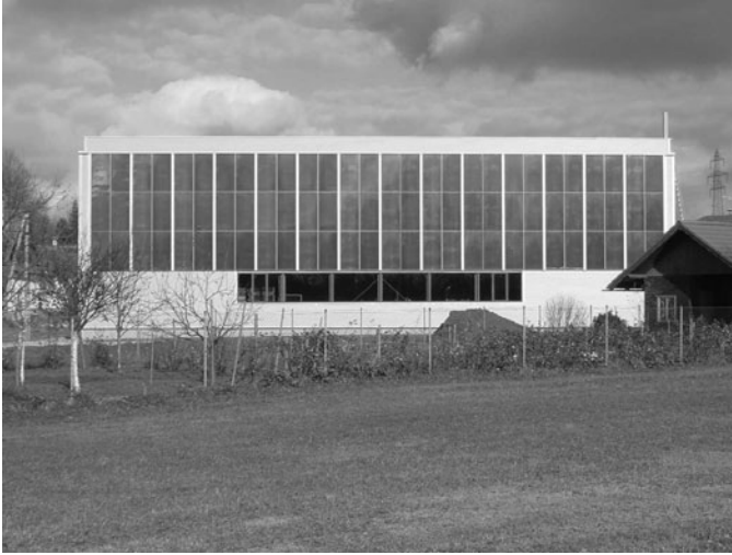
Figure 12.8 Example of a solar thermal collector system at a production hall in Tumeltsham, Upper Austria.
