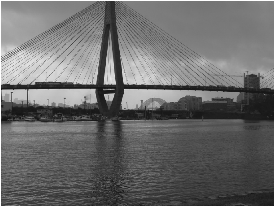
Figure 1.1 Sydney bridges. Photo S. Watson.
