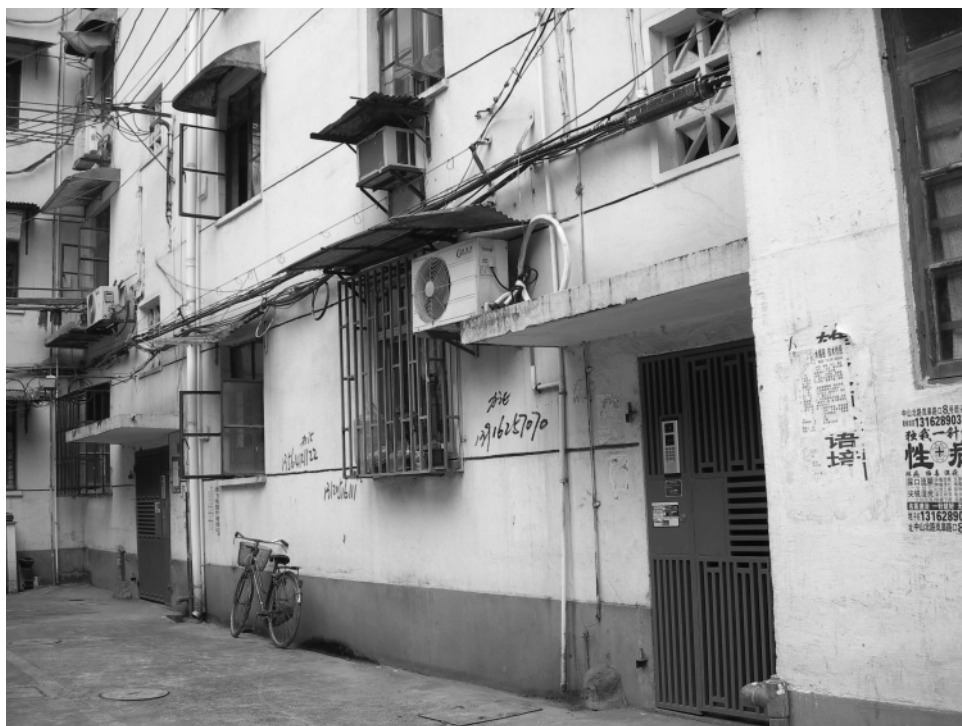
Figure 13.1 Entry door to privatized flat. Photo by Xiaohui Zhong.
