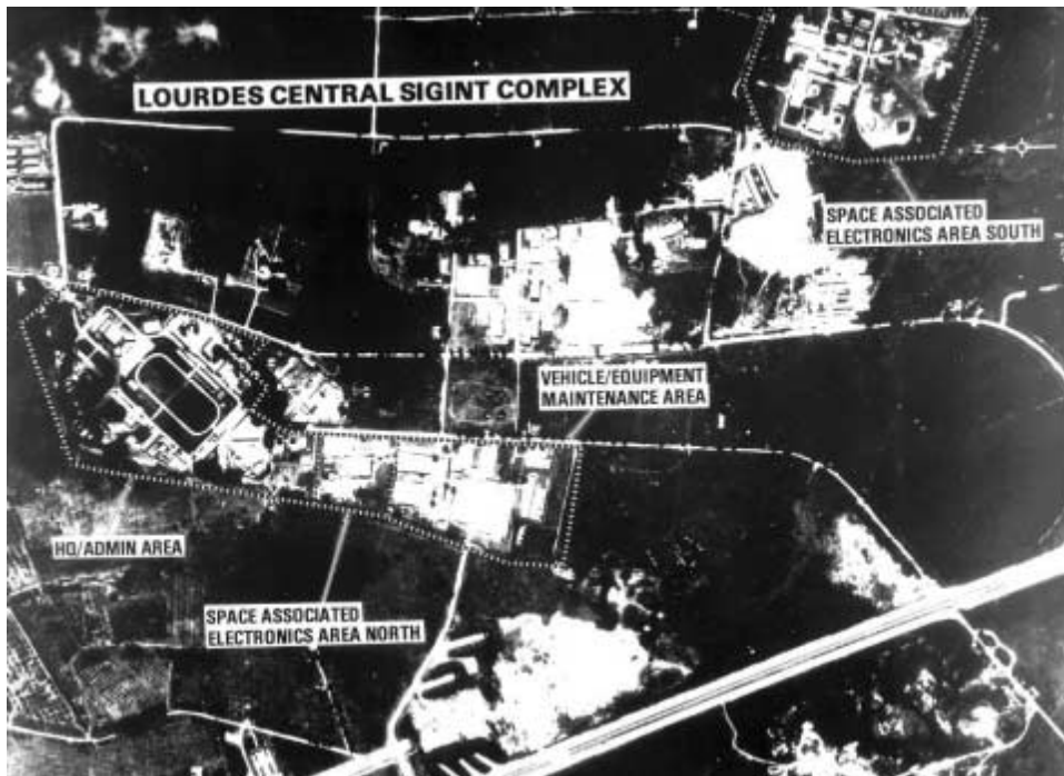
3-3 Lourdes signals intelligence facility located near Havana, Cuba.
