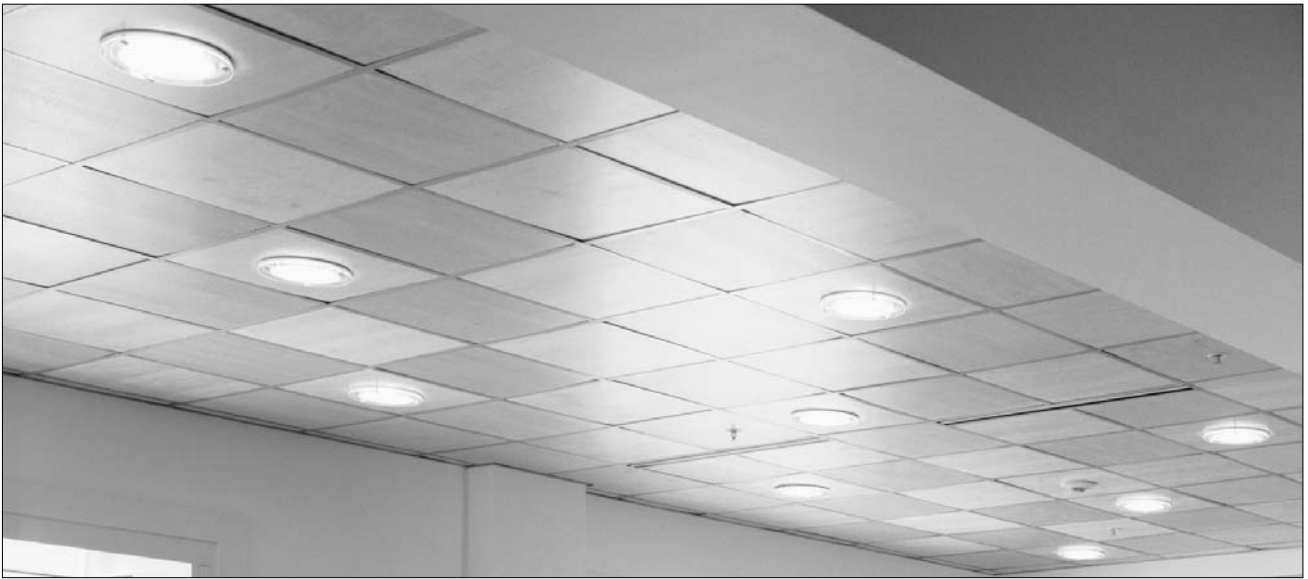
FIGURE 16-2 Many options for ceiling tiles are now available with high post-consumer recycled content, for either cellulose composition or mineral composition tiles.
