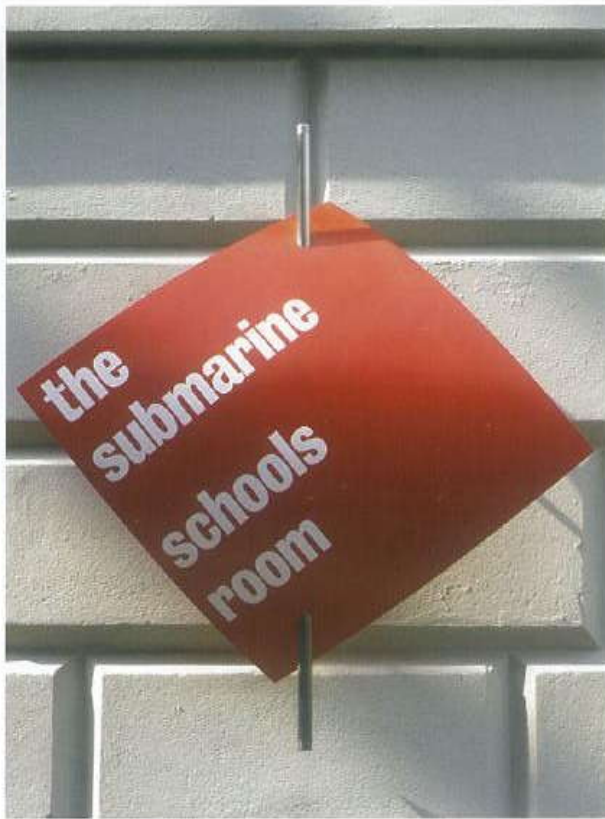
Left: The National Maritime Museum, London, internal signs. A simple sail and mast concept is a clever and appropriate design solution for a maritime museum. Note how the sign is held away from the brick work – a conventional flat wall-mounted sign would look 'stuck on' as an afterthought. The brightly coloured sails are easily spotted and the large type is very readable despite being on a curve. Design by Pentagram, UK
