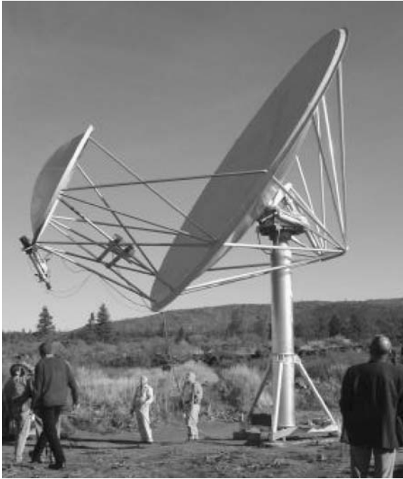
Figure 13. First ATA 6 m antenna assembly.
