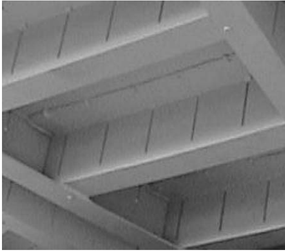
Figure 4. Hat and Z section framework holding back side of pie panel made with slat sheetmetal.
