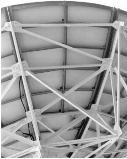
Figure 8. Dark members support panel surface; white members are reflector back structure frame.
