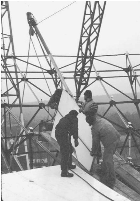
Figure 7. Panel size kept small for handling in light wind.
