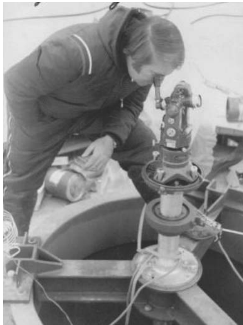
Figure 10. Theodolite used to set elevation angles to panel mounting clips and final alignment targets. Tape stretched to panel clip shown here.
