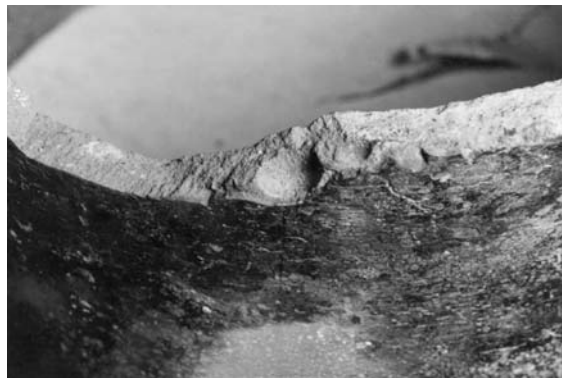
Figure 7.108 Circumferential failure of the pipe had originated at larger corrosion pit, and progressed in a brittle manner around the circumference in both directions
