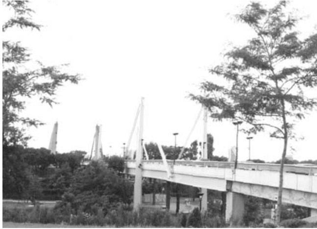
Figure 7.18 General view of the bridge 1
