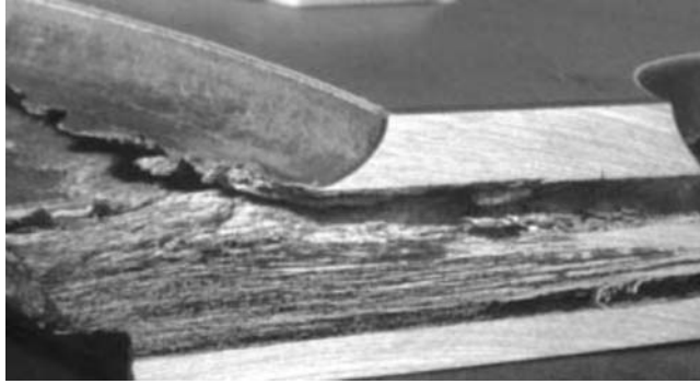
Figure 7.15 Cross-section through the panel, showing the exfoliation corrosion 1
