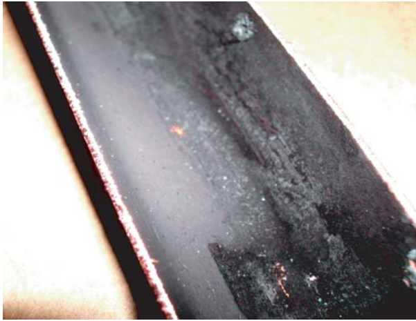
Plate 5 (Figure 7.56) Internal surface of pipe is coated with a thick, black, tightly adherent scale
