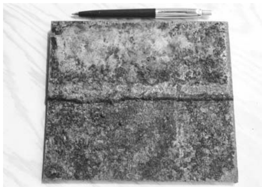
Figure 7.97 Plate 9 The inner surface of a steel plate cut from HRSG casing; note the rusty corrosion products and adhering insulation (top). (Reproduced from COM'1999 and 2005 with permission from the Metallurgy Society of CIM)
