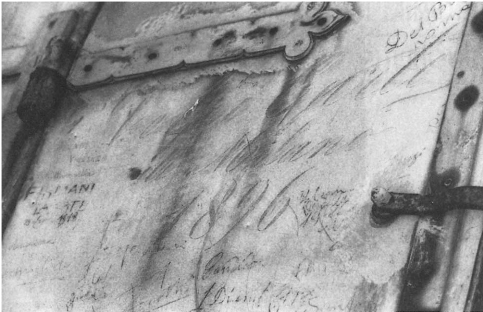
Figure C.5.2. Close-up view of the roof with steel hinges and graffiti.
