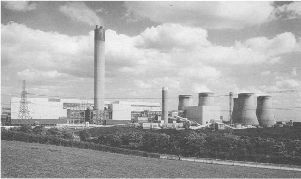
Figure 18.1 The FGD plant on Drax power station (courtesy National Power plc)
