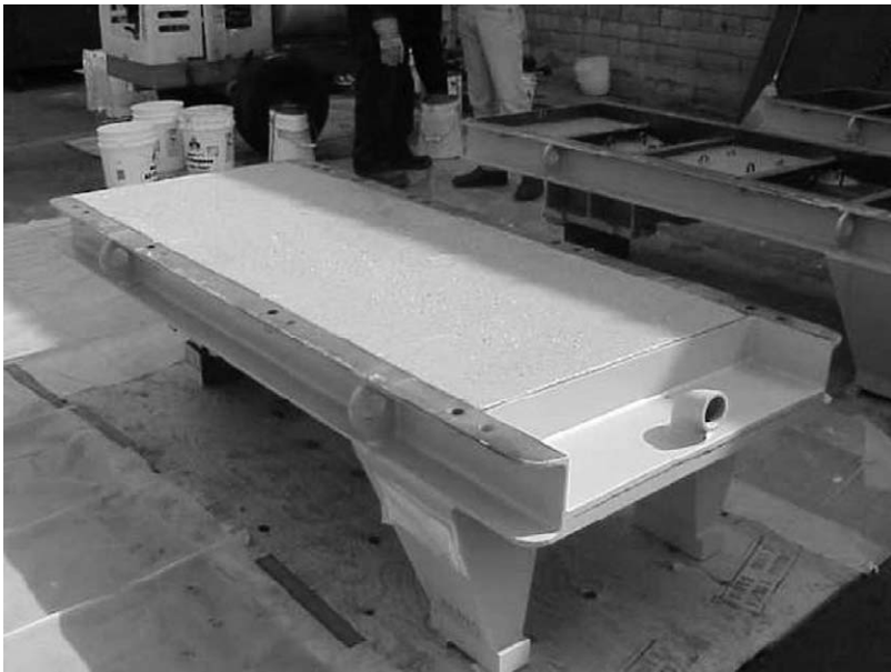
Figure 14-14. Pre-grouted pump base (bottom view).
