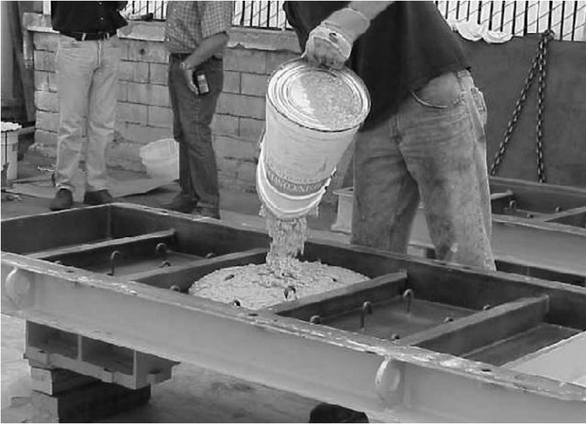
Figure 14-13. Pre-grouting a pump base.
