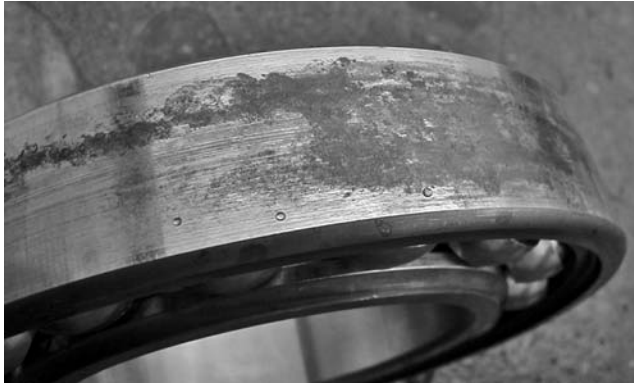
PHOTO 10.9 This dark discoloration is “fretting”.
