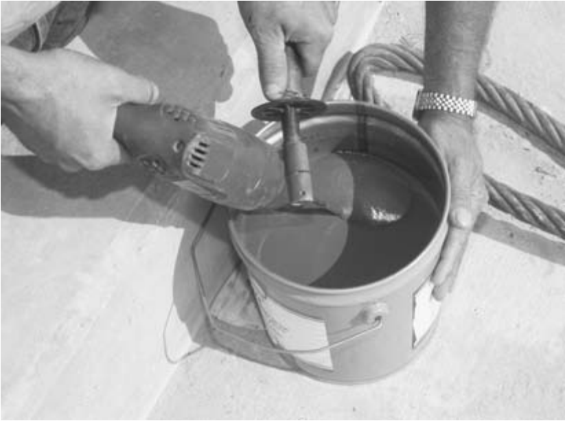
Figure 3-47. Mixing of low viscosity epoxy grout.
