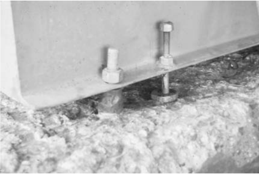
Figure 3-36. Anchor bolt and jack bolt system.
