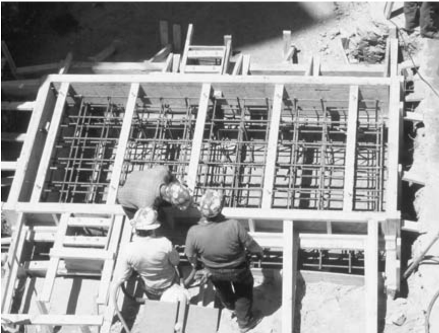
Figure 3-27. Construction of machinery foundation.
