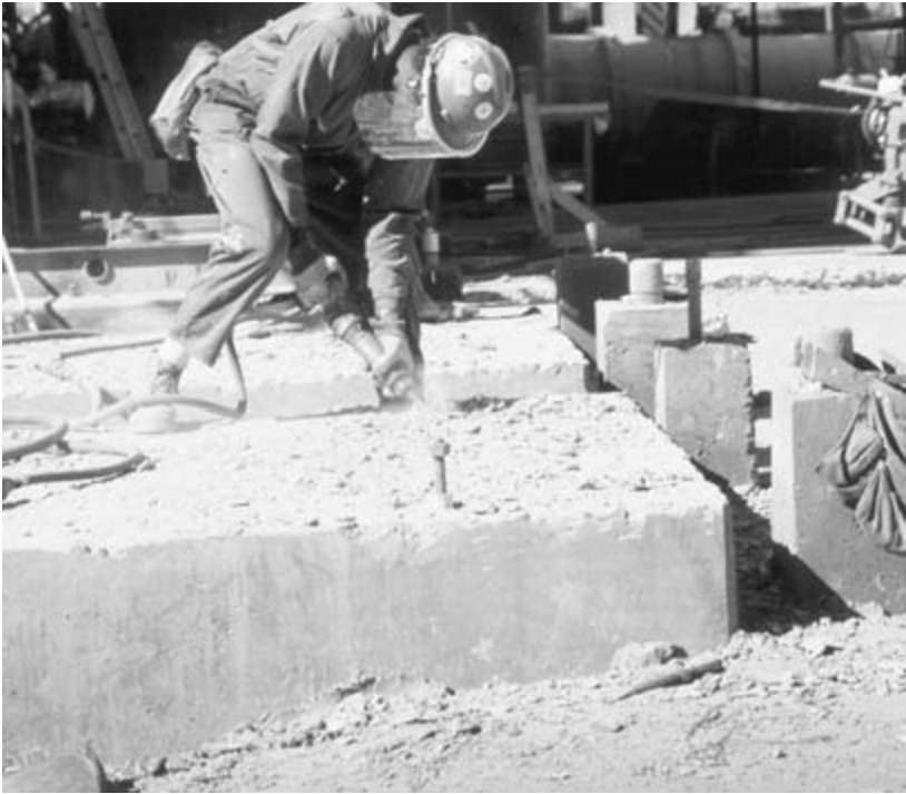
Figure 3-48. Chipping of concrete foundation.
