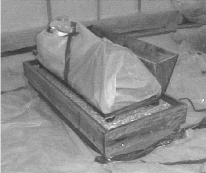
Figure 3-45. Pregrout installation using conventional method.
