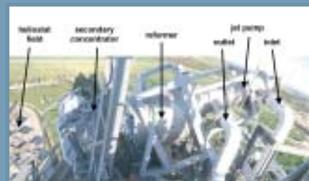
The state-of-the-art reformer on the WIS Solar Tower in Israel.
