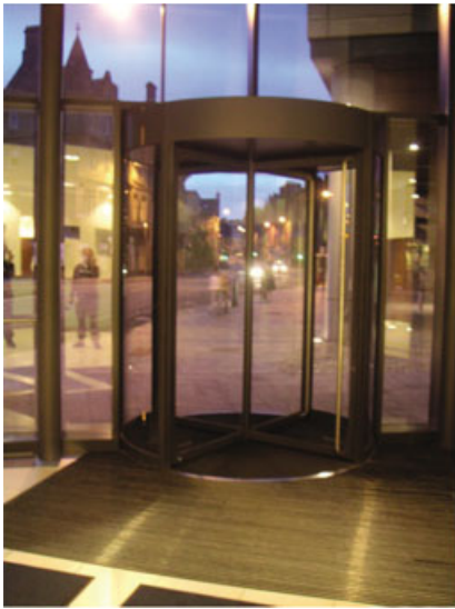
Figure T12.5 Checking for seals on doors to stop heat loss
