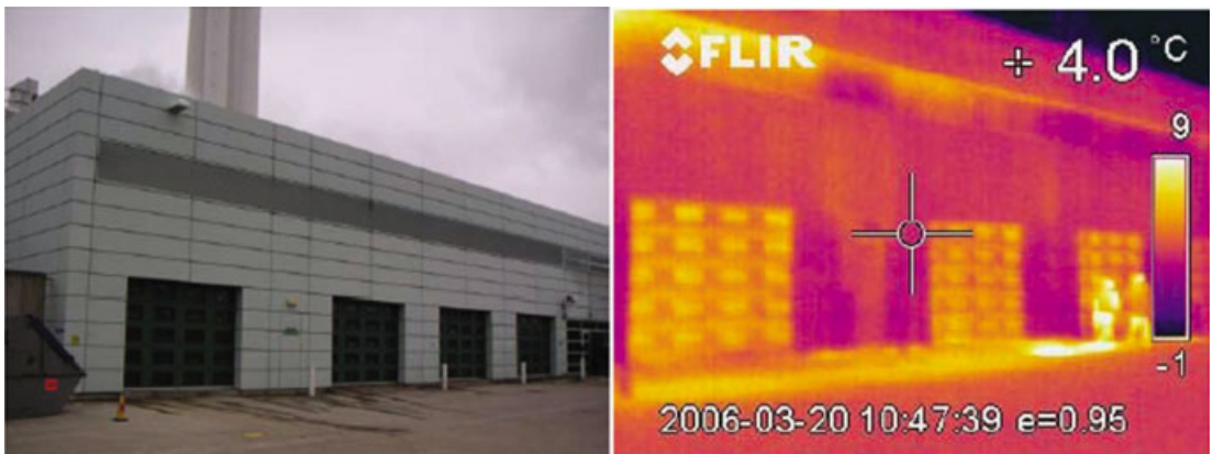
Figure T12.1 Survey of building fabric
