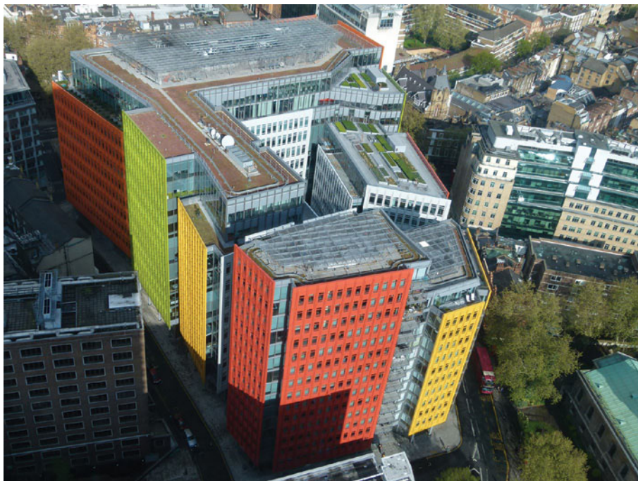
Figure 2.3 Retrofit and refurbishment will be key in making an impact
