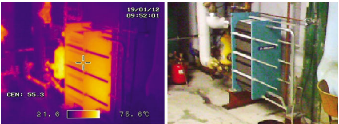
Figure T12.19 Heat exchanger uninsulated
