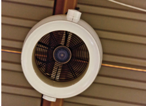
Figure 9.4 De-stratification fans
