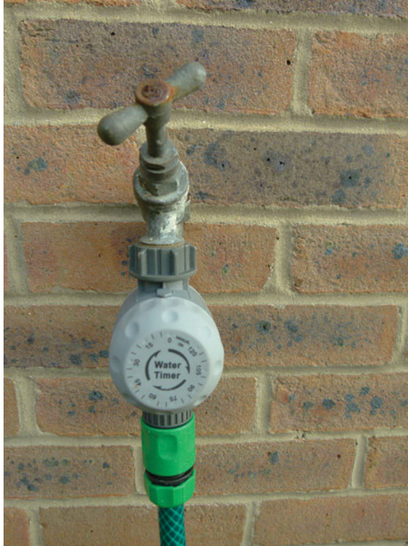
Figure 7.10 A simple 'clockwork' water timer
