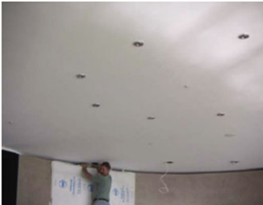
Figure T12.6 Behind the plasterboard ceiling reveals chilled ceiling
