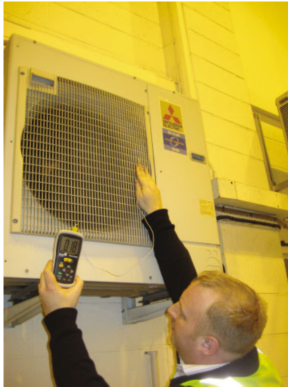
Figure 12.5 Measuring temperature performance and efficiency
