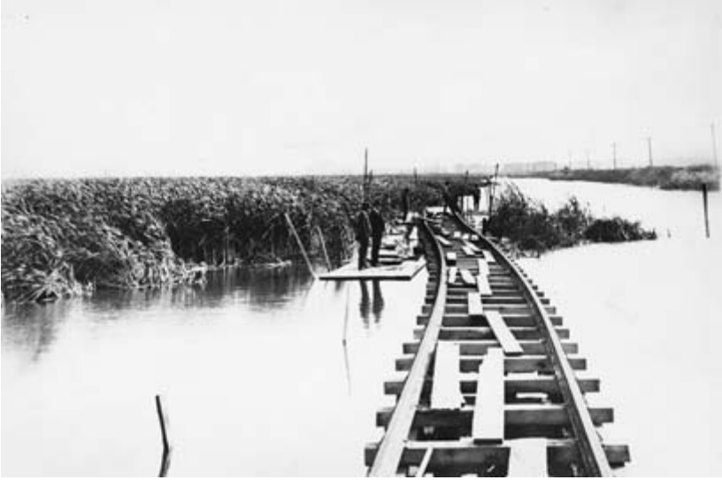
18. Laying streetcar track across Hyde Lake in 1915. Courtesy of the Southeast Chicago Historical Museum.
