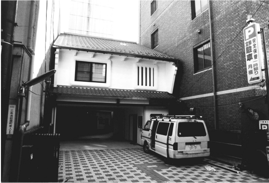
Figure 9.6 Kyō-machiya -style second floor over parking-tower drive-through.
