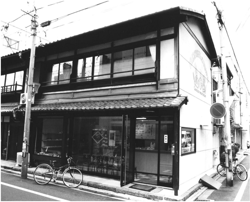
Figure 9.4 Renovated kyō-machiya pastry shop with glass front.
