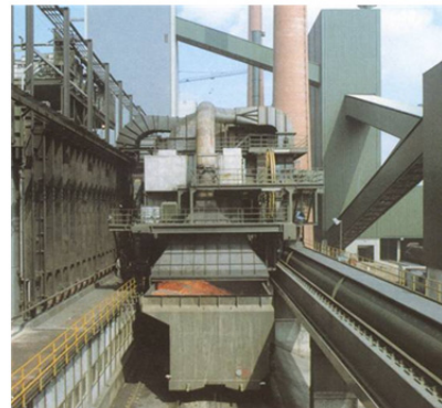
Figure 18. Coke pushing without (left side) and with coke side dedusting (Coking Plant Prosper, Germany - right side)
