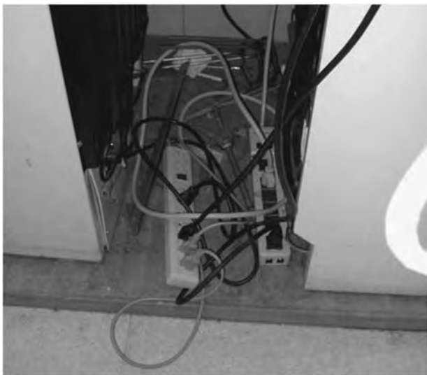
FIGURE 5.3.5.3 Outlets Clustered on Floor. It is common to use electrical strips since there are often multiple modules of an instrument(s) that need to have electricity. It is easy to forget that plugging in lots of equipment into these electrical strips could present a fire hazard. If the numerous cords are not neatly contained they can present other hazards such as trip hazards or shock hazards if a water spill enters into the strip.
