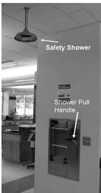
FIGURE 2.1.3.2 A Laboratory Safety Shower. It is very important to know the locations of the nearest safety showers in laboratories or in nearby hallways. During an emergency, time is critical.
