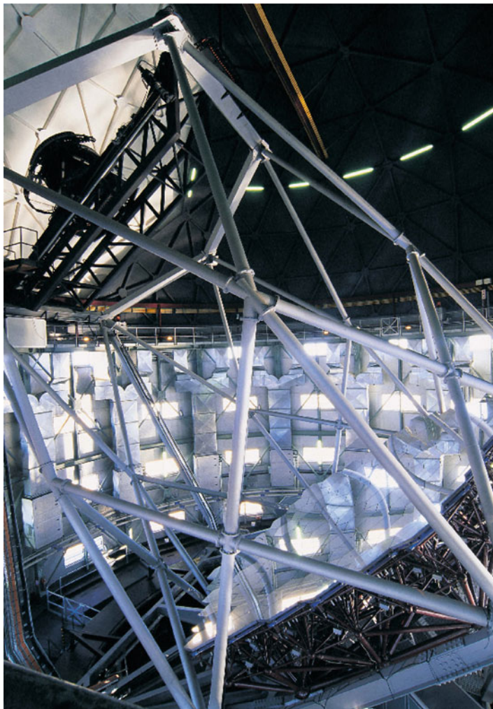
Fig. 12.5 SALT, as completed in 2005, showing the primary mirror array, its mirror support truss, and the dome louvres open. At top is the Tracker, which carries the SAC (Spherical Aberration Corrector) and instrument payload
